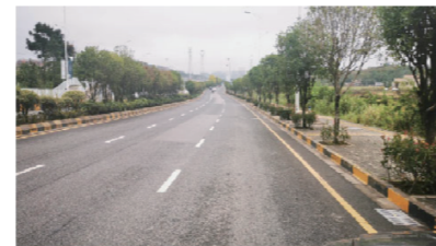
Mixed road surfaces
