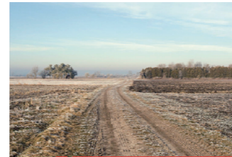
Poor unpaved road surface
