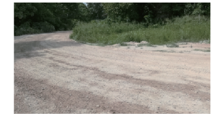
Mixed road surfaces
